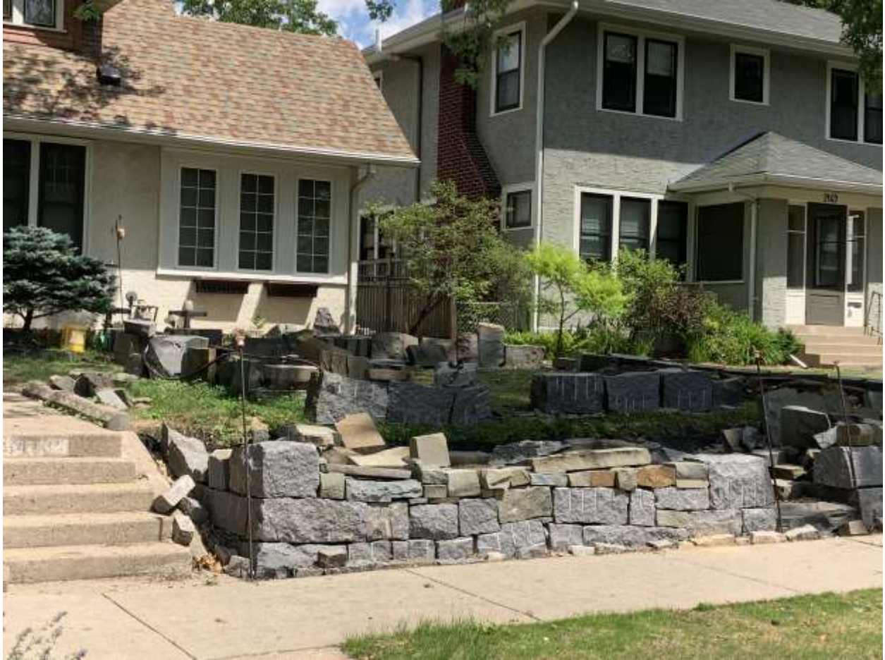
1473 Fairmount Ave. Retaining Wall 7-7-26
