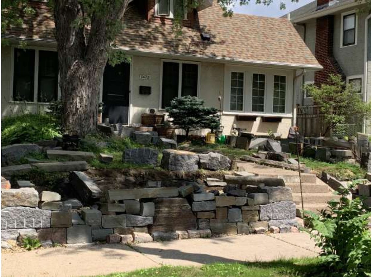
1473 Fairmount Ave. Retaining Wall 7-7-26
