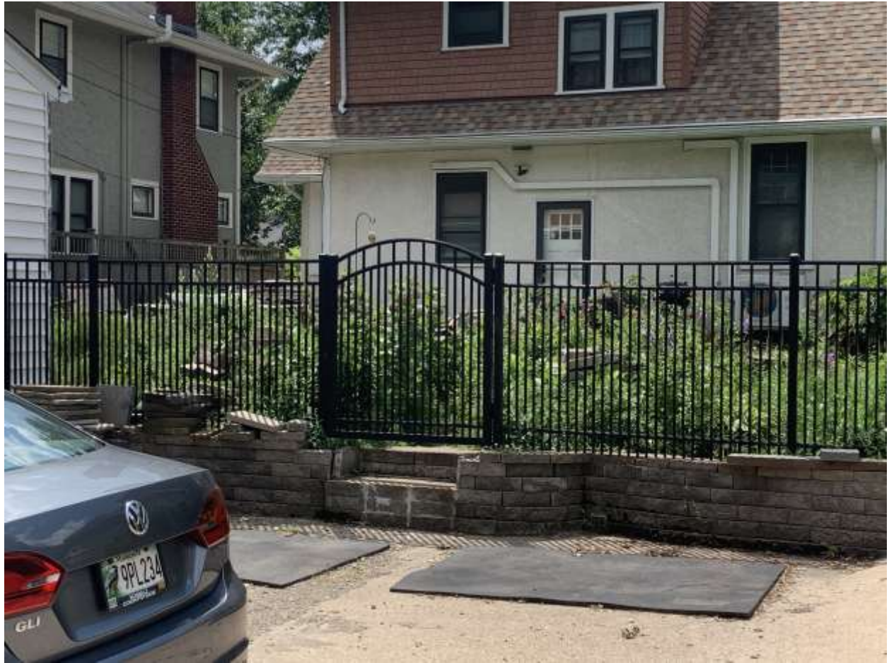
1473 Fairmount Ave. Retaining Wall 7-7-26
