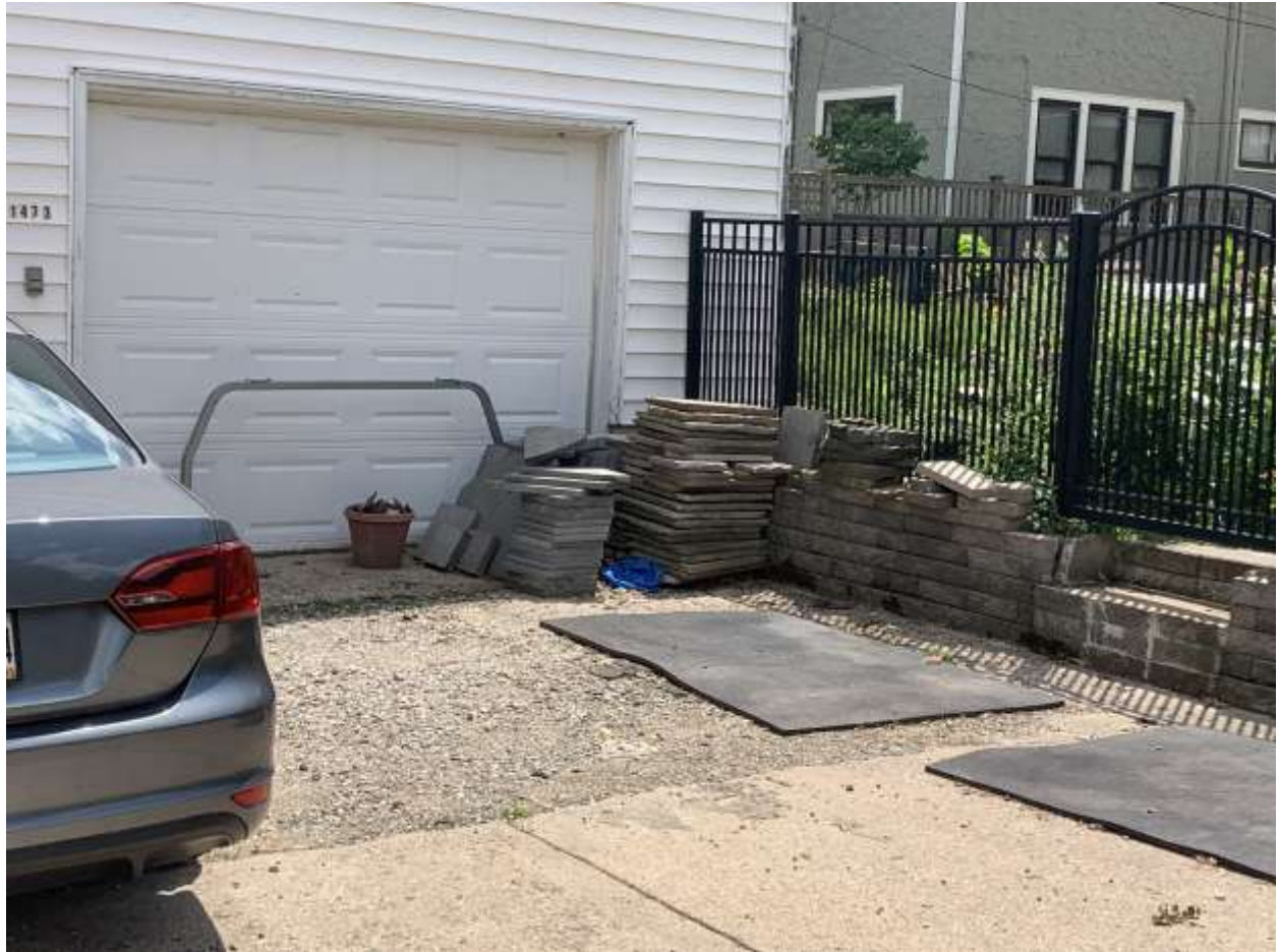
1473 Fairmount Ave. Retaining Wall 7-7-26
